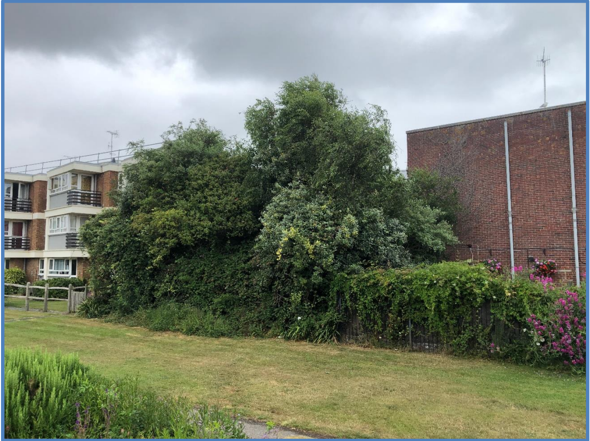
PLATE 5-2: VIEW OF THE DEVELOPMENT AREA FROM THE SOUTH-WEST
