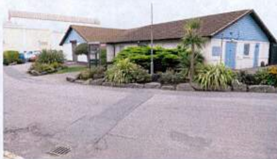
01 – Existing Building pictured from NW
