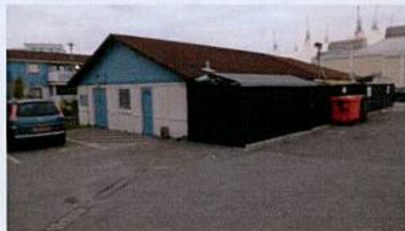
02 – Existing Building pictured from SW
