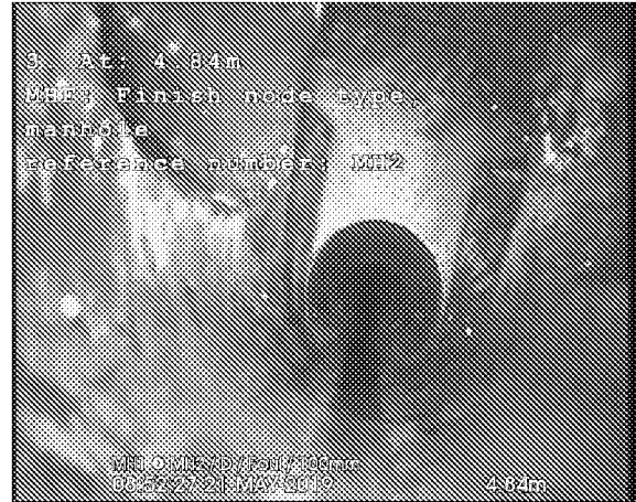
190521_0852A-Survey.jpg, 00:00:42, 4.84 m Finish node type, manhole, reference number: MH2
