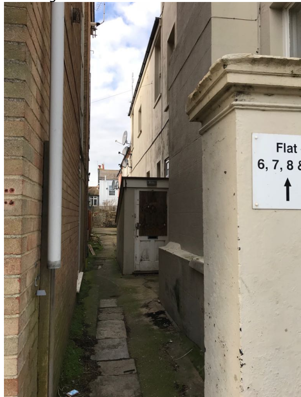
View of side passage from Steyne Gardens/ Flat 6 External entrance
