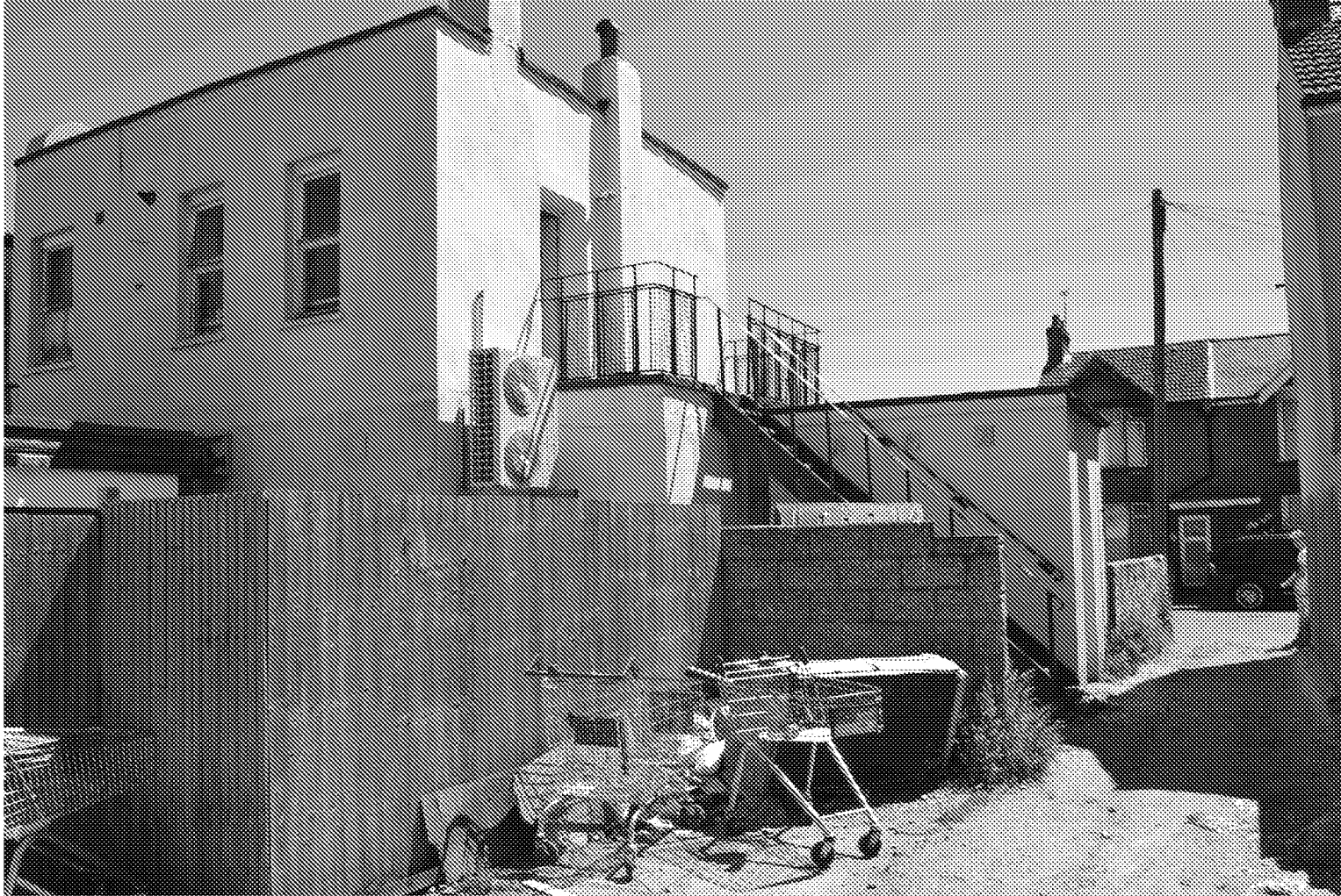
PHOTO 2 SHOWING REAR OF 11a STATION ROAD WITH EXISTING SINGLE STOREY EXTENSION, ACCESS ROAD AND TIMBER STAIRS UP TO FIRST FLOOR
