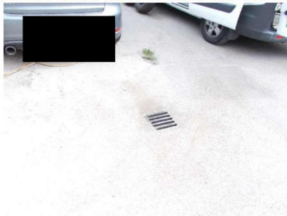
Surface water drain in the front forecourt of the nursery building
