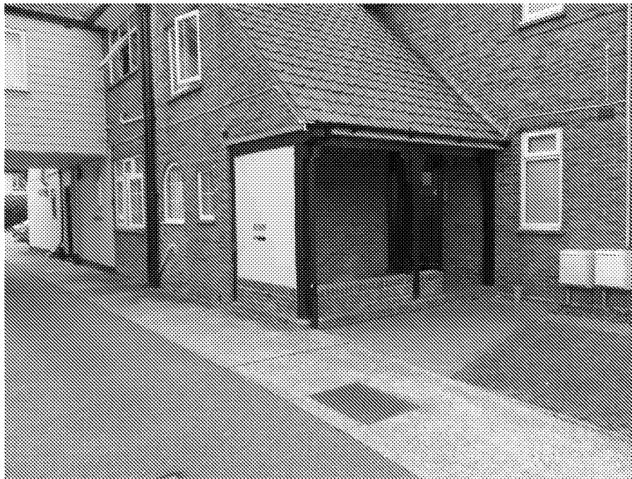
5 – Porch to the converted to Bin Store
