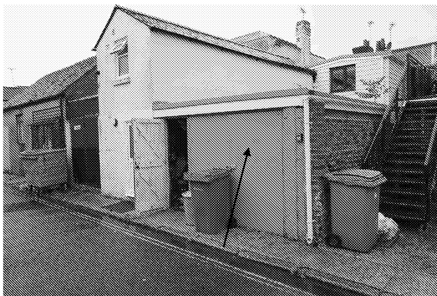
Fig.3: View of the garage at rear of No.21 from Sadler Street (Grey doors)
