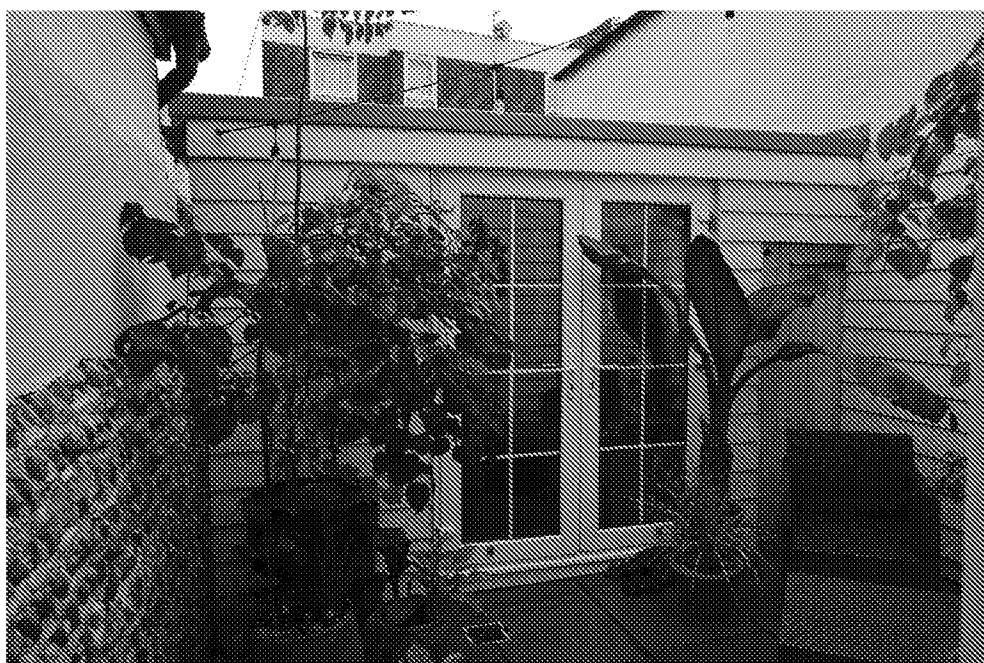
Fig 5: Part view inside the attractive courtyard of No. 21 looking east. Double doors to be replaced by single door.
