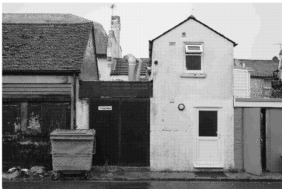
Fig 4: View from Sadler Street showing existing roof lines.
