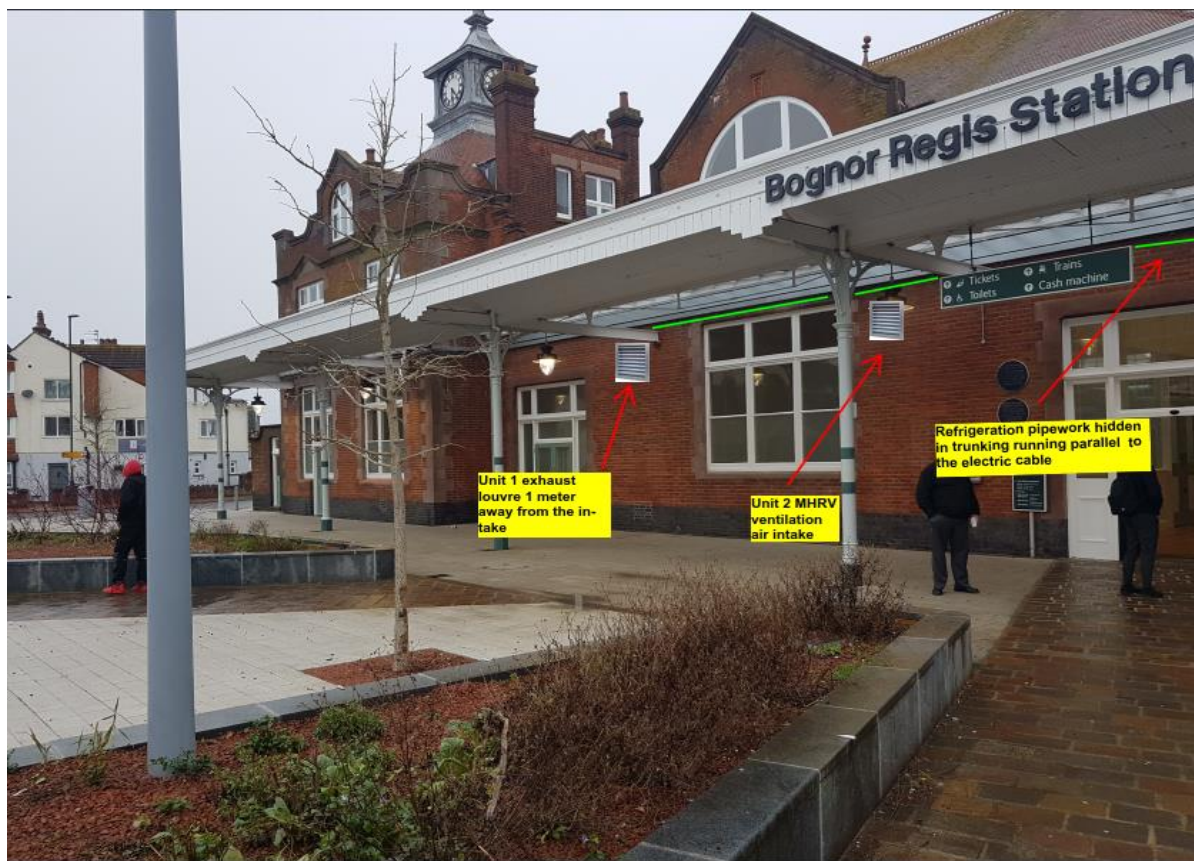
Figure 3 : External louvre MHRV proposed location for unit 1
