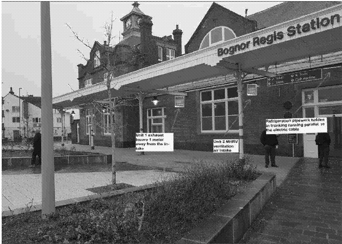
Figure 3 : External louvre MHRV proposed location for unit 1
