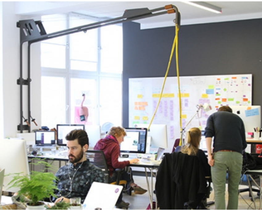
And boom with suspended power leads for tables in the middle of the floor. With the boom connected to the underside of the mezzanine.
