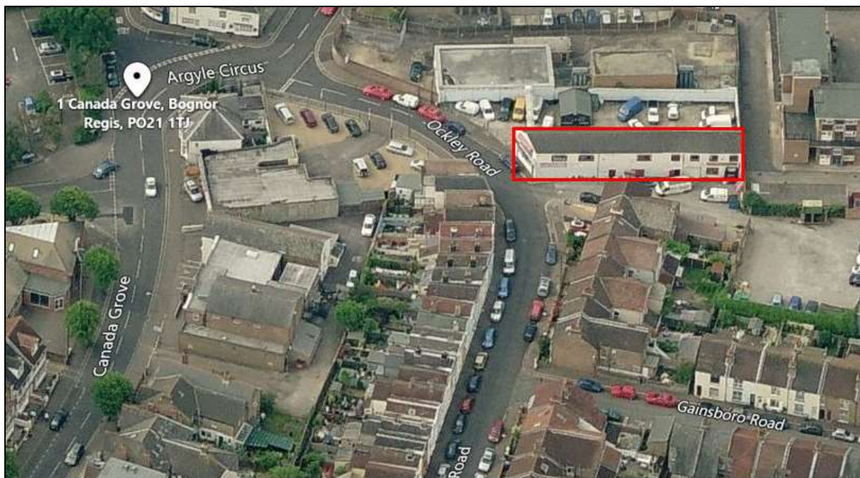
Figure 1. Aerial Image of the site with the site shown in red
