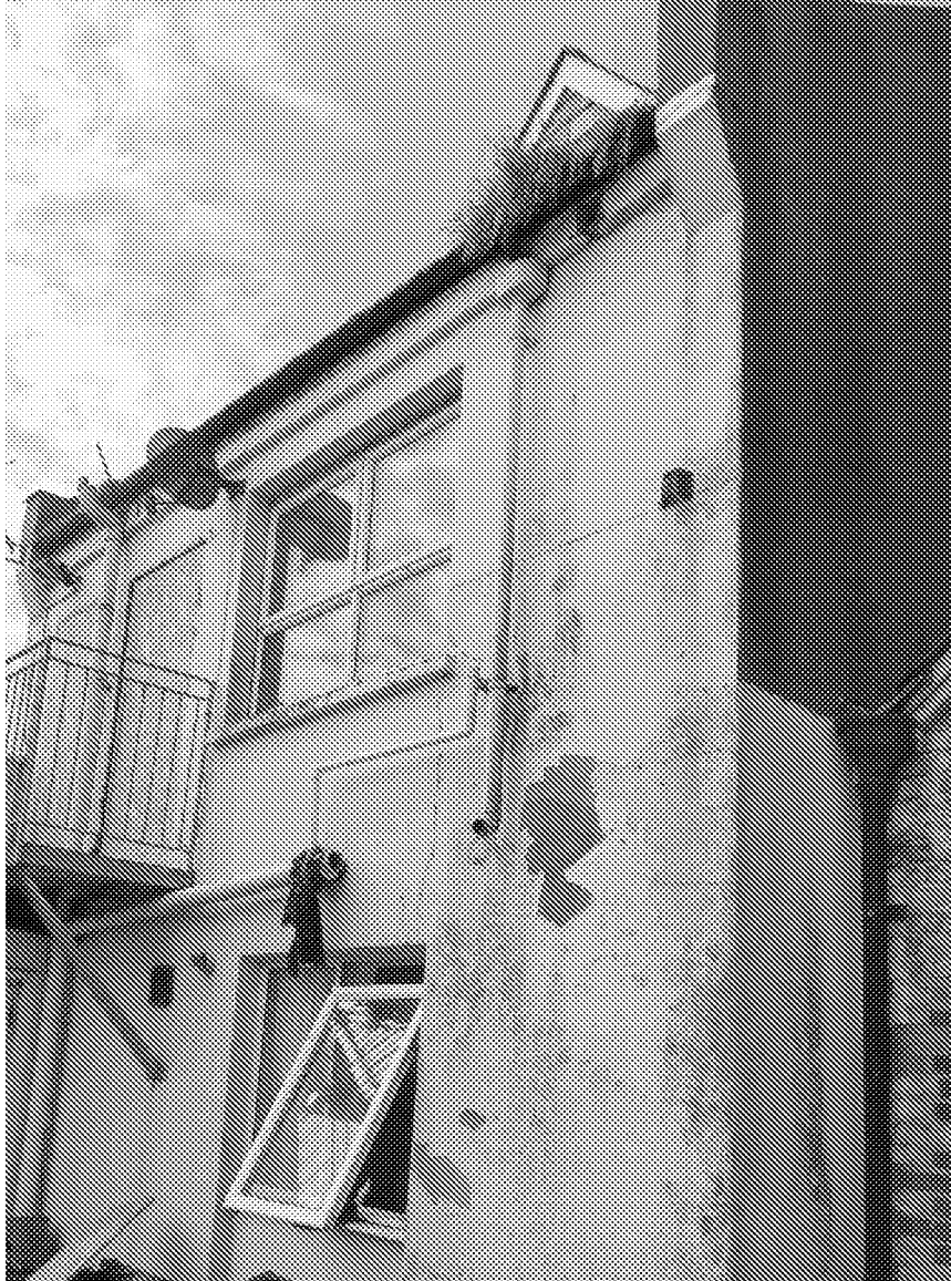
Image 7 & 8 – Extensive cracking to rear first floor render (So will need to be removed to find hidden issues and enable any repair) Erosion of mortar joints, with many soft joints requiring repair (This lets water into the structure and corrodes many other elements lower down)
