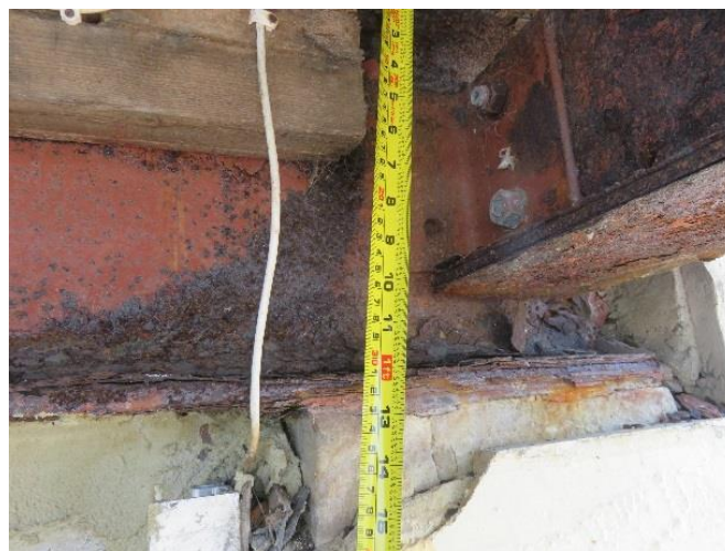
Image 6 - Waterloo Square Elevation – Severely laminated balcony steelwork support beam left and right hand end respectively
