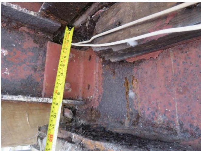
Image 6 - Waterloo Square Elevation – Severely laminated balcony steelwork support beam left and right hand end respectively
