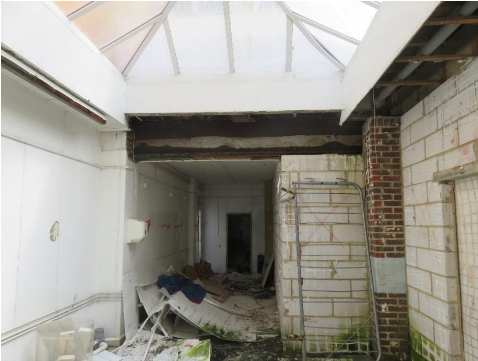
Image 1 – Overall View of Beam
