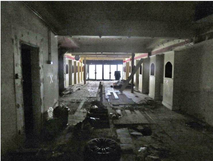
P15 –Abandoned internal works No. 2 Waterloo Sq.
