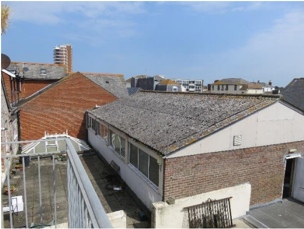
P2 - View of Gym Structure (First Floor)
