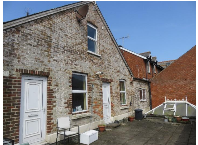
P8 – Access to 1st Floor Flats Norfolk Street
