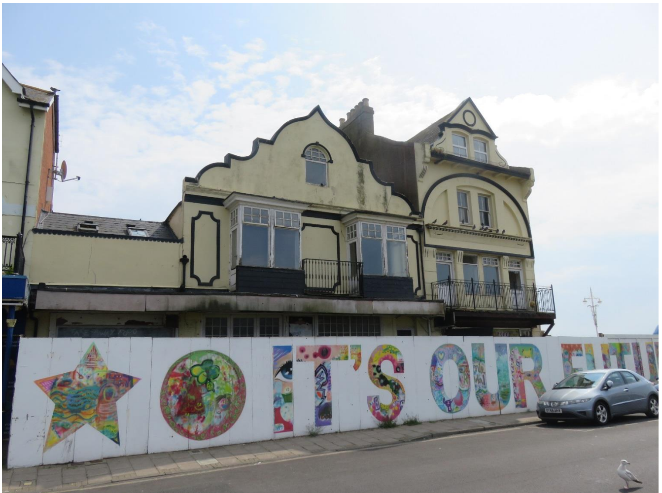
P1 - Waterloo Square View
