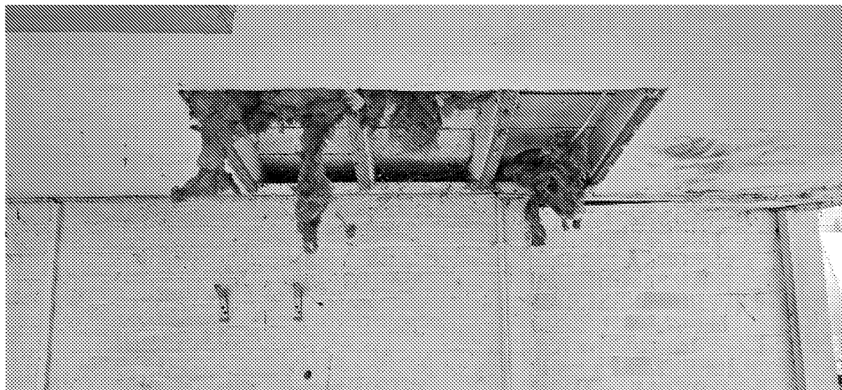
Photo 7 – Internal east wall of the storeroom with visible age to the plasterboard and insulation within this section of the building
