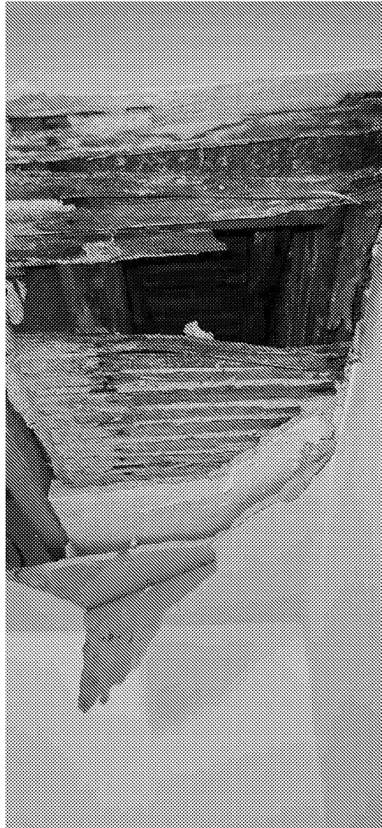
Photo 10 – Damaged lath and plaster of the ceiling in the rear of the commercial space
