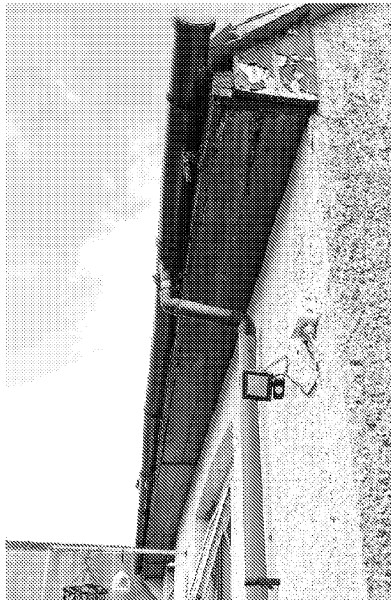
Photo 6 – Timber soffit box on the back of the main roof highlighting gaps in the soffit and fascia
