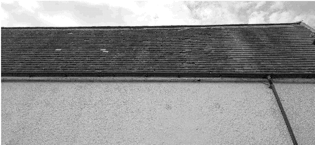
Photo 4 – Neighbouring property bordering the rear, southern, boundary. Multiple hanging tiles with gaps from missing or broken tiles
