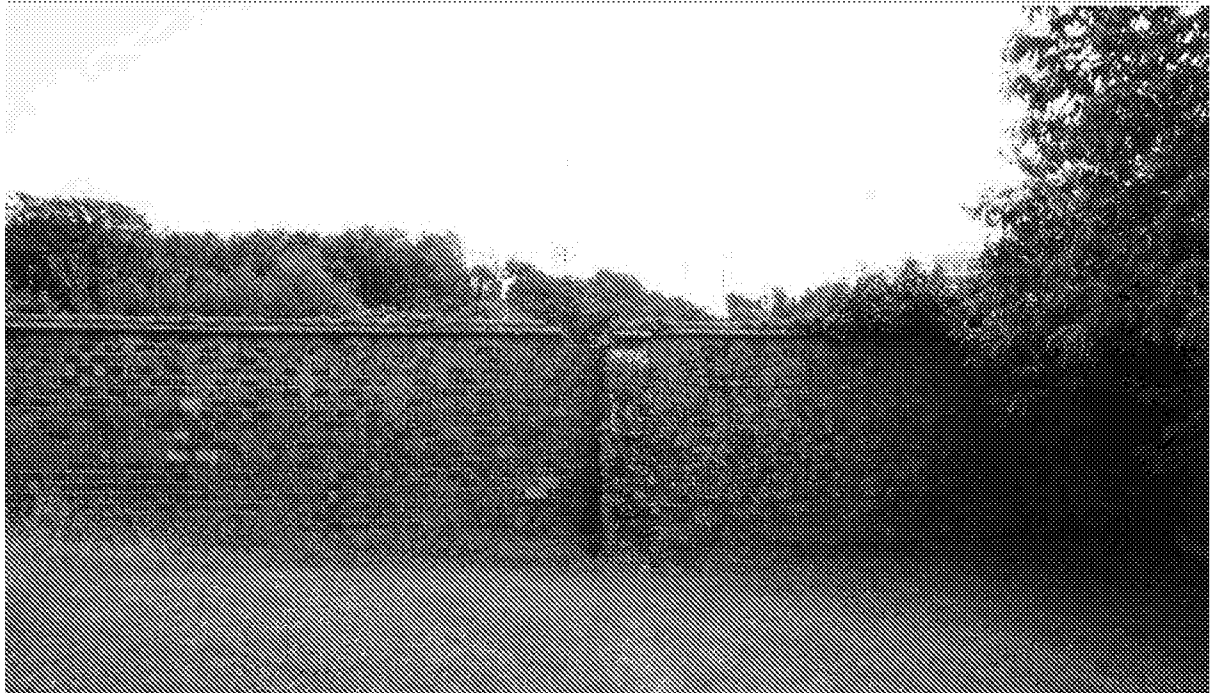
Figure 13: East boundary wall to No.71 Upper Bognor Road (to north of serpentine wall)
