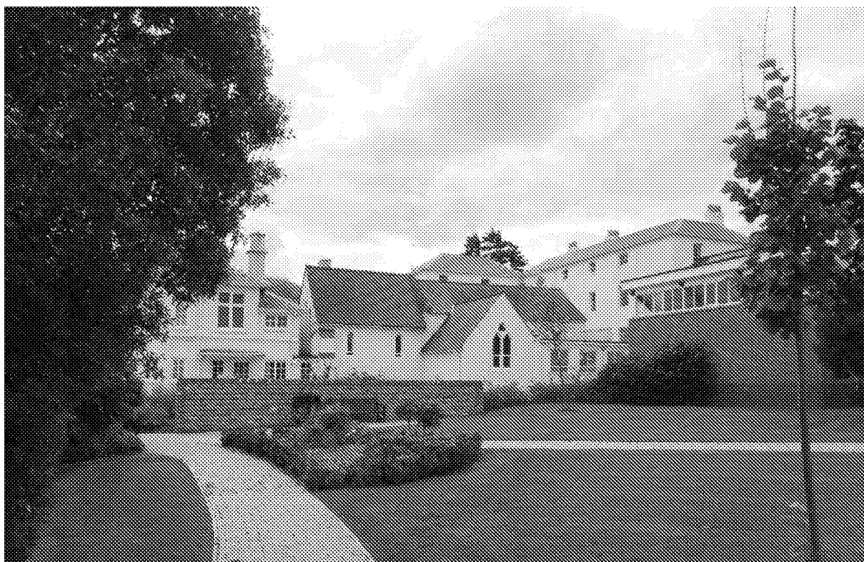
Figure 4: No.57 St Michael's House, Upper Bognor Road – chapel and north elevation
