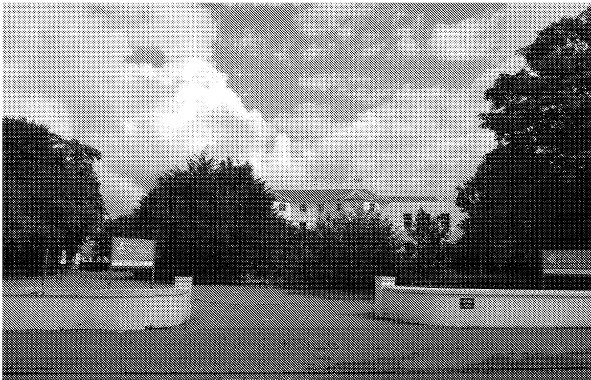
Figure 25: View looking north from Upper Bognor Road - main entrance to campus
