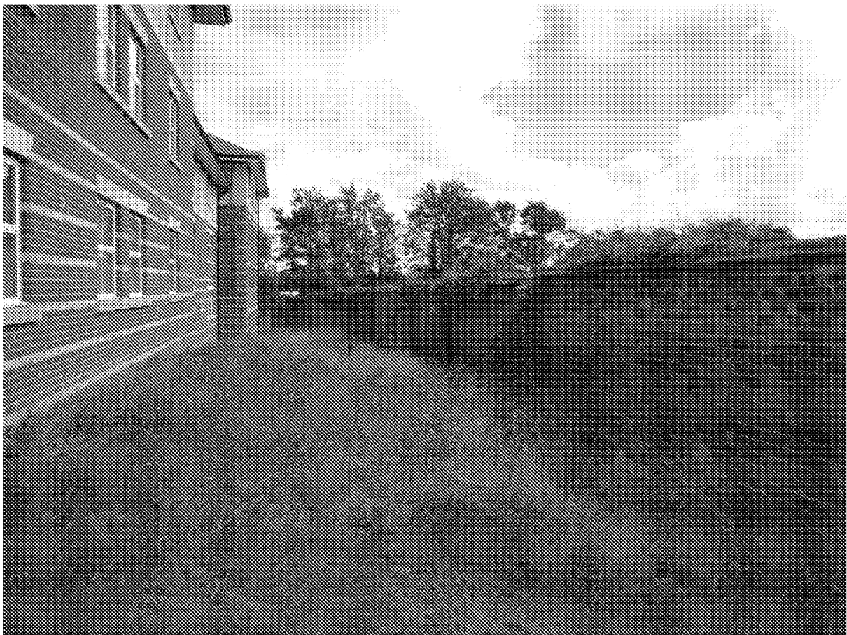
Figure 14: Eastern boundary wall to the east side of Barbara Smith Halls
