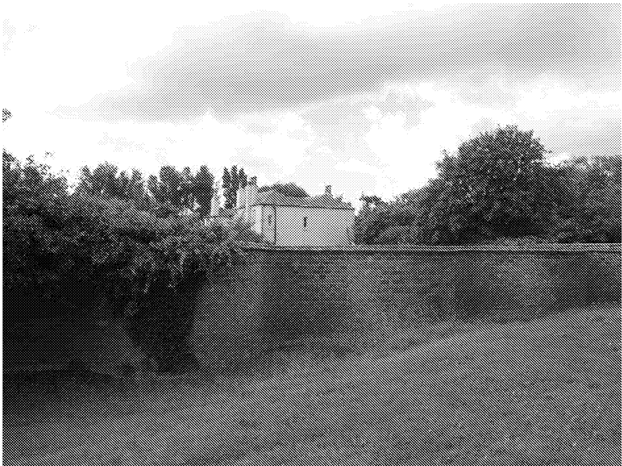
Figure 12: Serpentine wall (north elevation) No.71 Upper Bognor Road beyond
