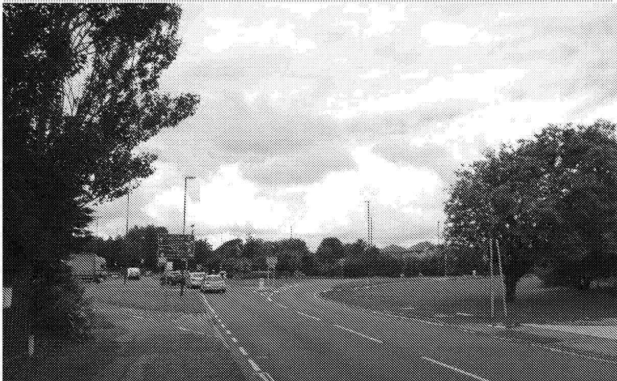
Figure 21: View towards the western boundary of the conservation area
