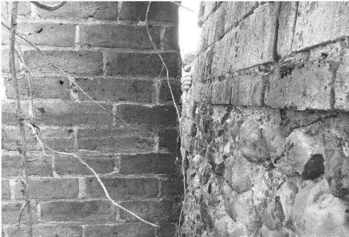
Figure 20: Brickwork of woodstore/outbuildings relating to existing wall
