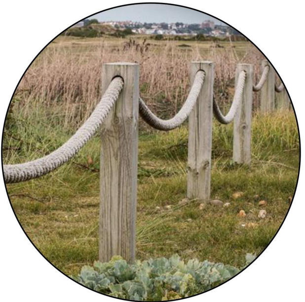
Barriers Fixed bollards with rope in-between
