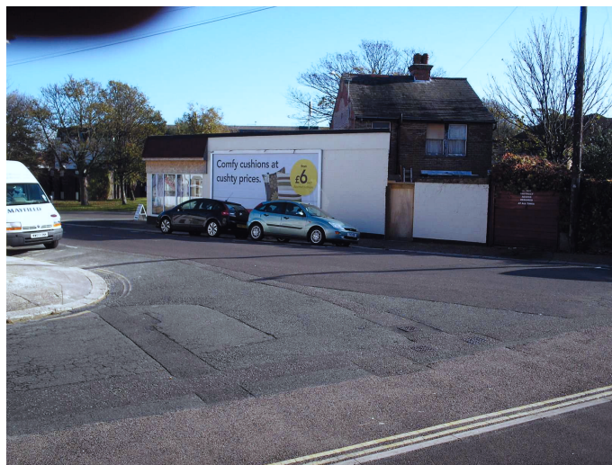
Site from Spencer Street
