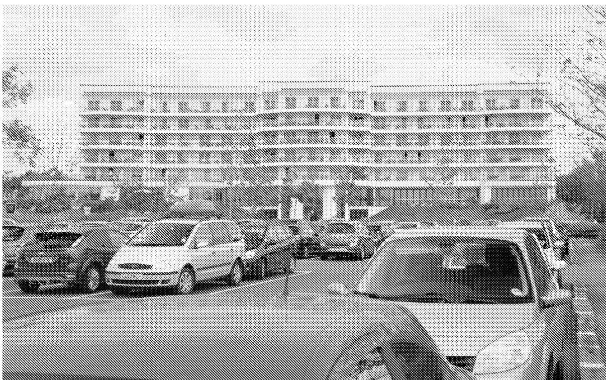
Photograph facing north at the proposed location with the Ocean Hotel in the background
