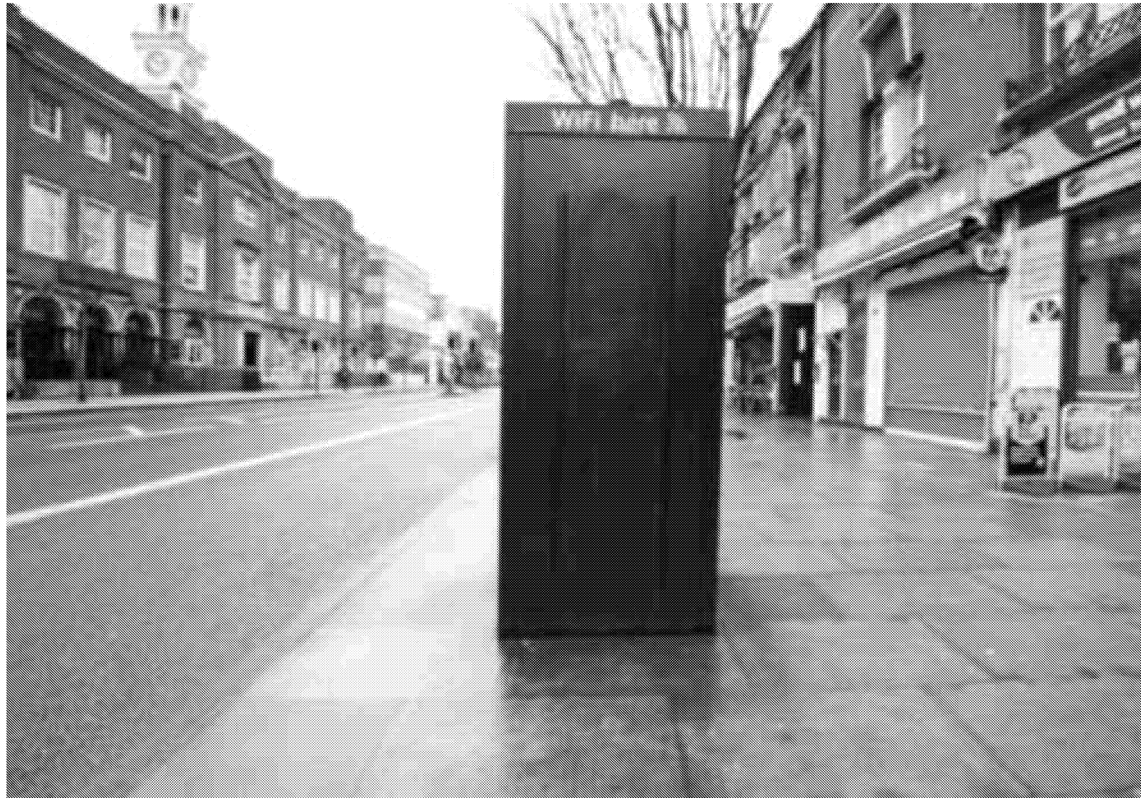
Existing Telephone kiosk
