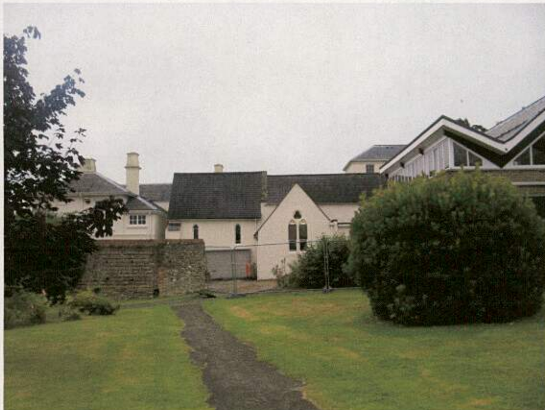
The historic wall before it blew down in a gale, November 2011.
