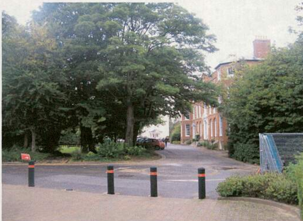
The Dome Frontage in 2012, which shows dense tree cover and parking to the front.
