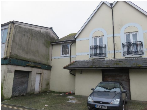
Norfolk Street view of the rear of the building
