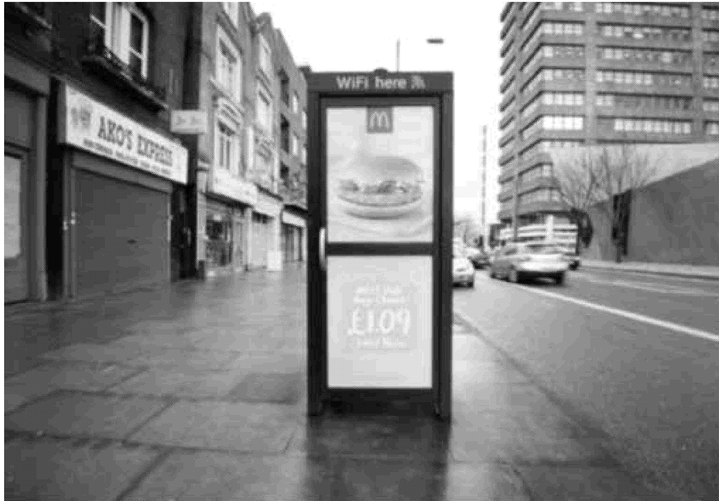
Existing Telephone kiosk
