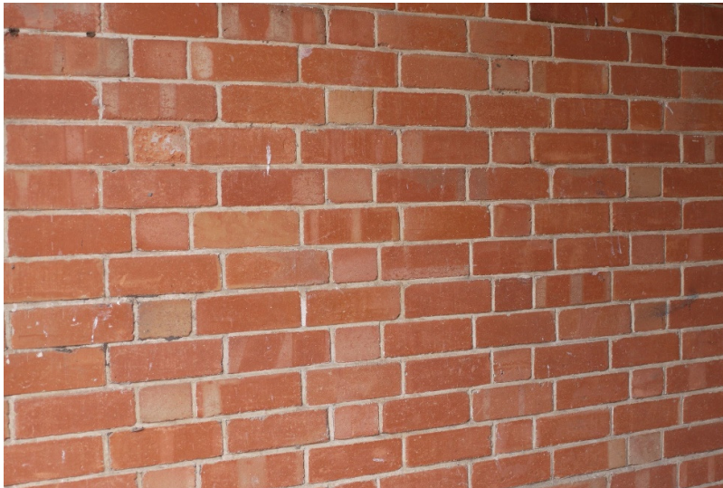
Picture – Example of 'Sussex' or 'Flemish Garden Wall' bond brickwork.
