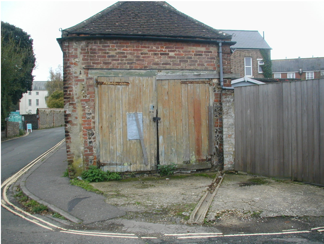
Photo – Existing garage wall elevation.
