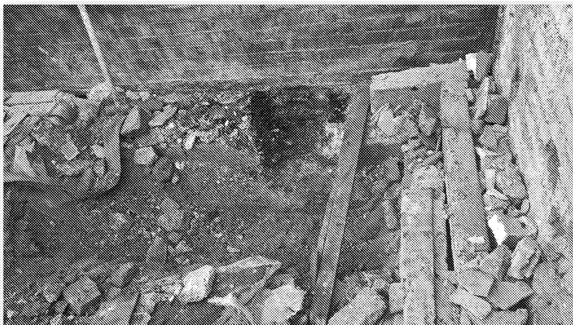
Photograph 3 – More complete removal of floor slab and exposure of building foundation
