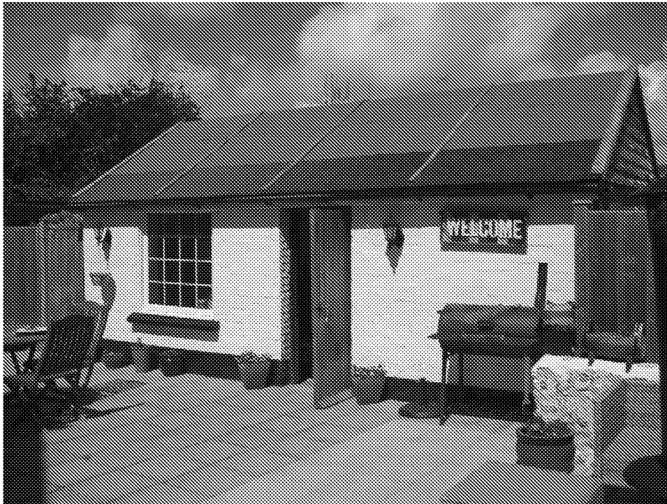
Photograph 1. Side elevation of the existing garage (Southern elevation).
