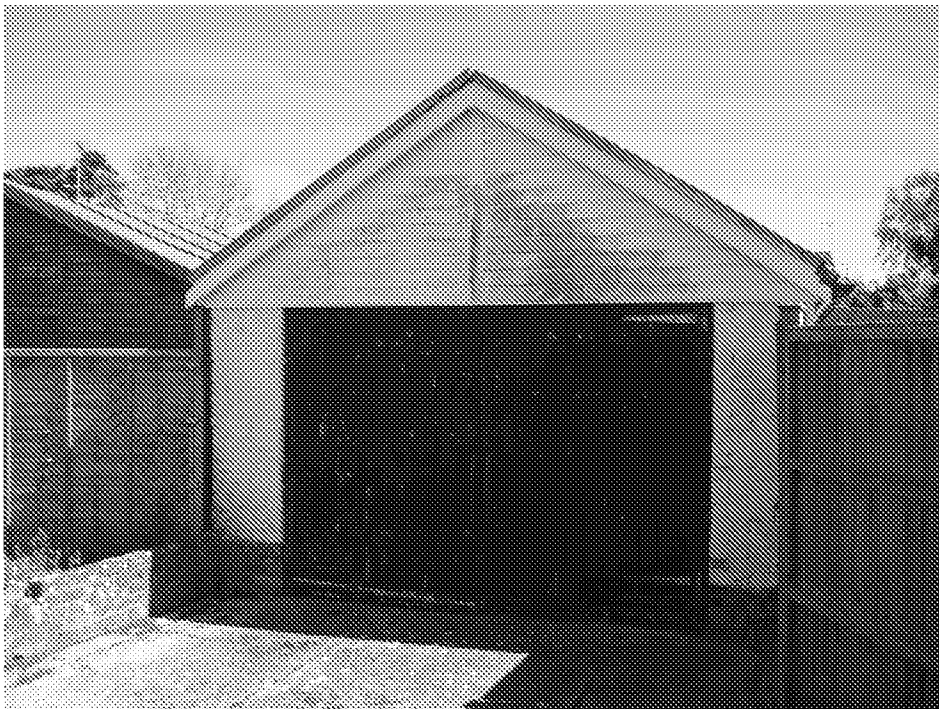
Photograph 2. Front elevation of the garage (Western elevation).
