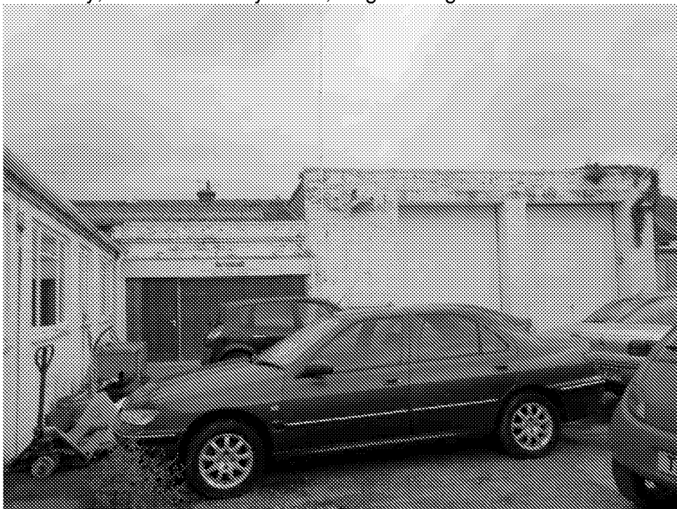
Photograph 2.2: Buildings utilised as mechanical workshops along the northern site boundary, Land off Ockley Road, Bognor Regis.
