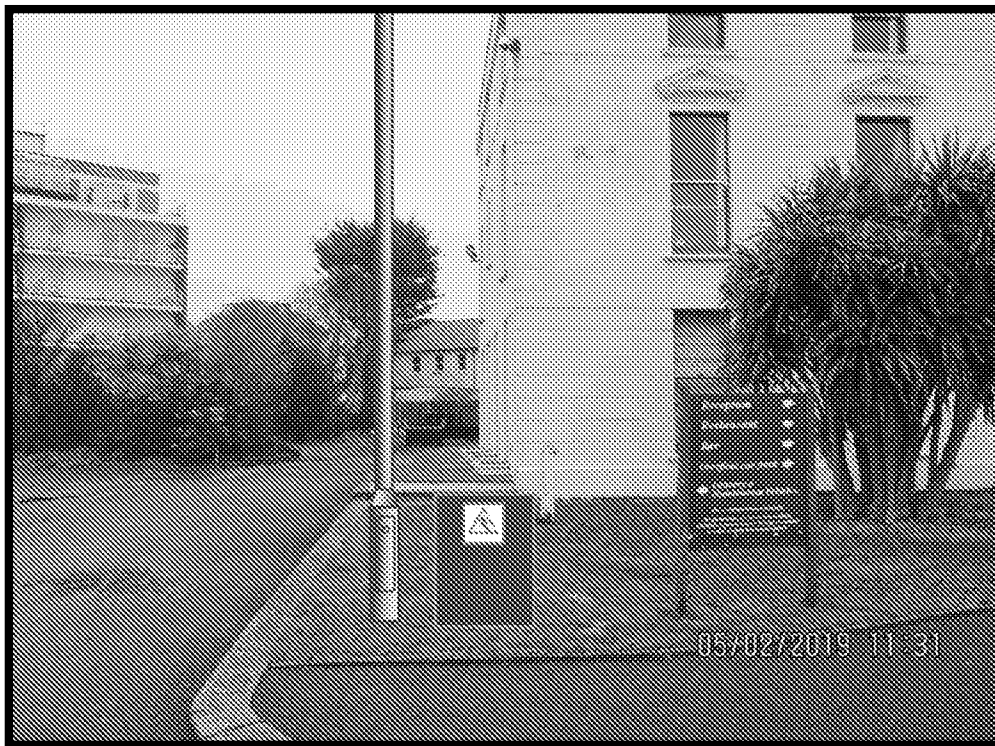
Location 1 (Showing External Cabinet)
