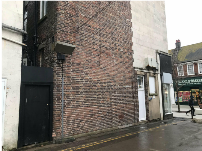
3. Existing Buildings ,Looking North-East
