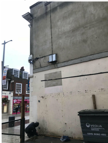
7. Existing Buildings ,Looking East
