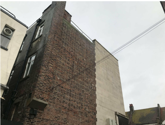
5. Existing Buildings ,Looking West
