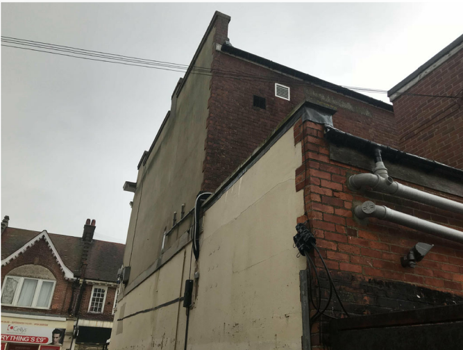
2. Existing Buildings, Looking South-East
