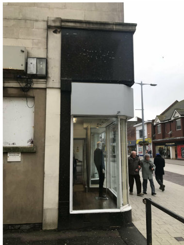
4. Existing Buildings , Looking to London Road
