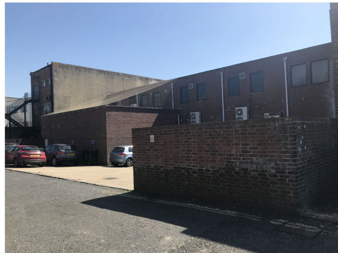
4. Bedford Street ,main acces
