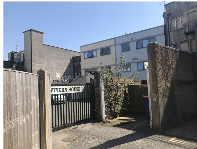
6. Bedford Street ,main acces
