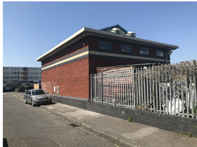
7. Bedford Street ,main acces
