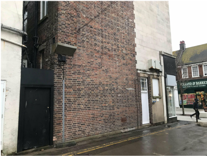
3. Existing Buildings ,Looking North-East
