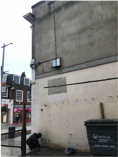
7. Existing Buildings ,Looking East
