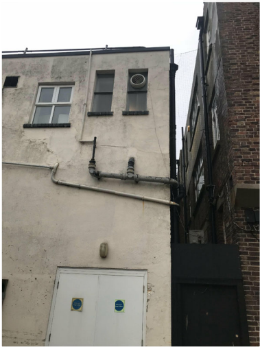
1. Existing Buildings, Looking North
