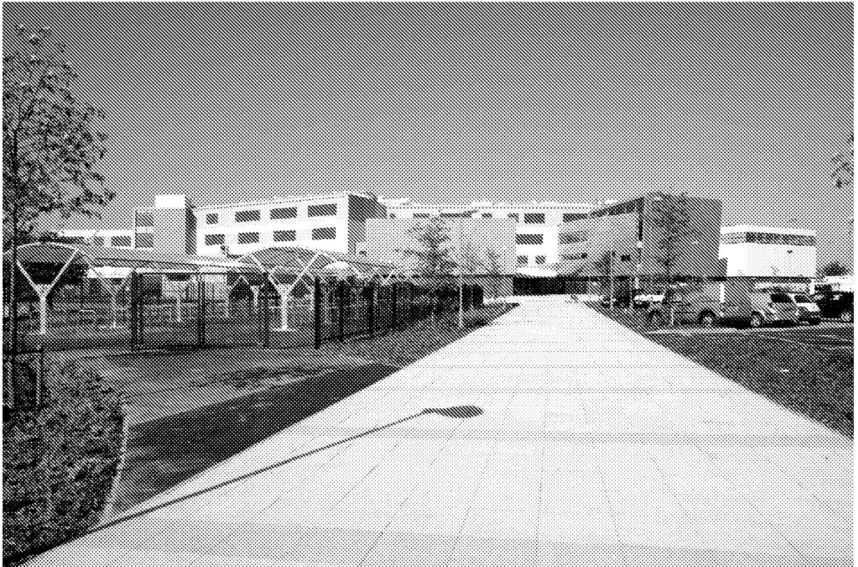
Entrance to the school with the energy centre behind the cycle store to the left
