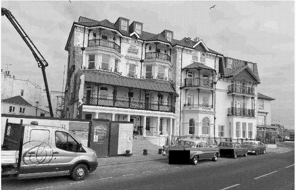
Photo 2: Current refurbished Royal Hotel. The Jack Rabbit Slims portion has been demolished.
