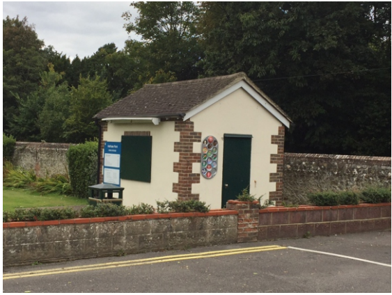
VIEW A EXISTING HUT TO BE CONVERTED INTO TOILET AMENITIES
