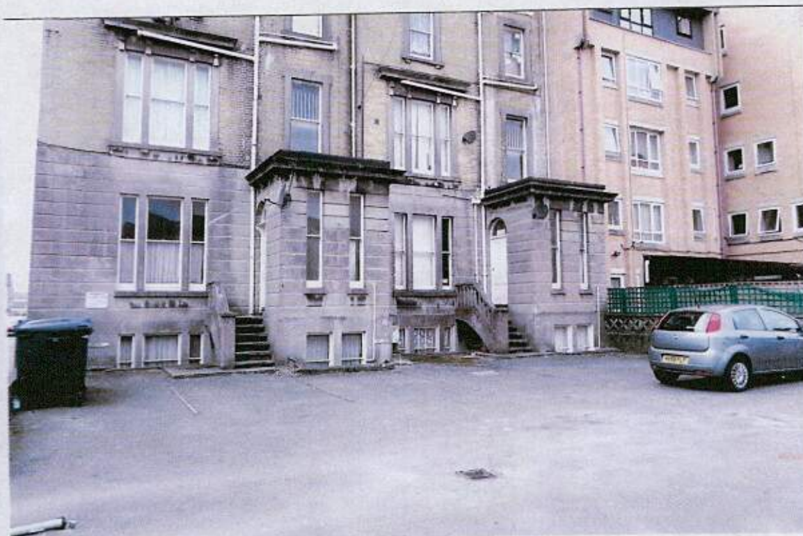
View of rear of existing flats/offices and car parking area.
