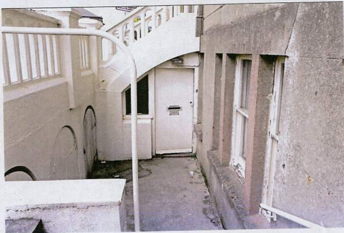
View of office entrance off Clarence Road at lower ground floor.
