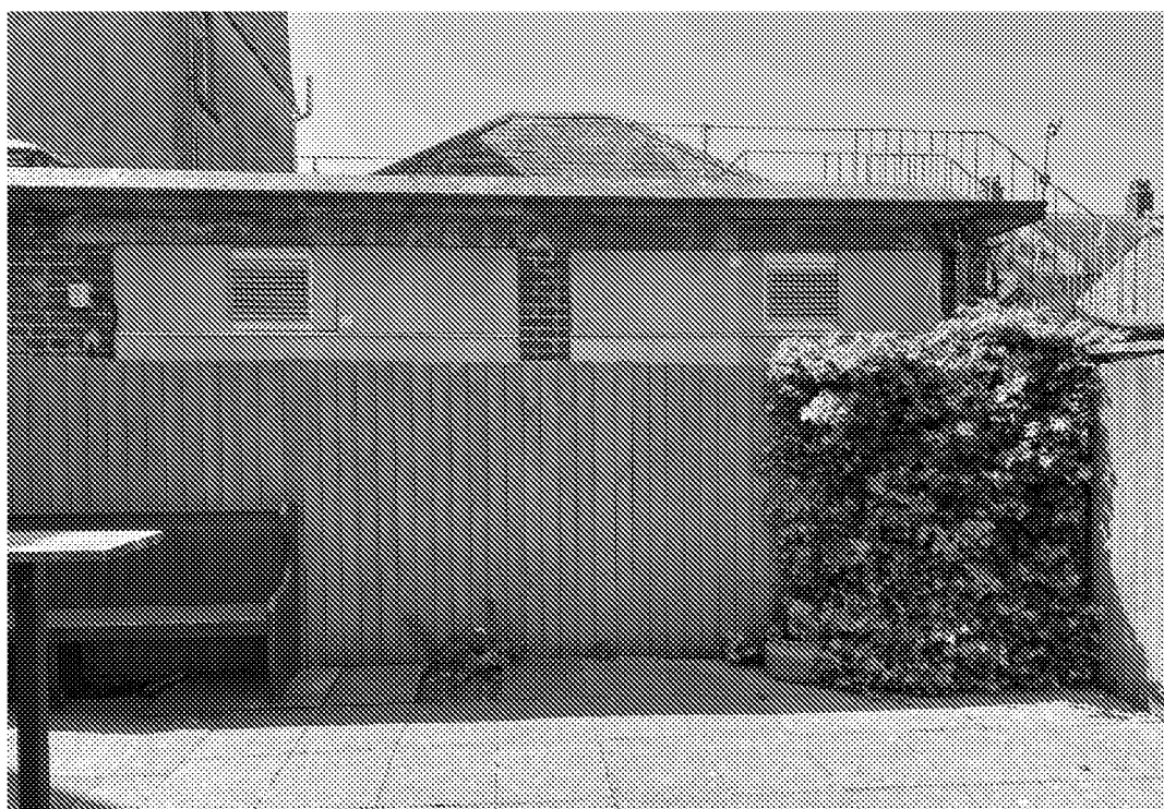
Image showing existing back of house area
