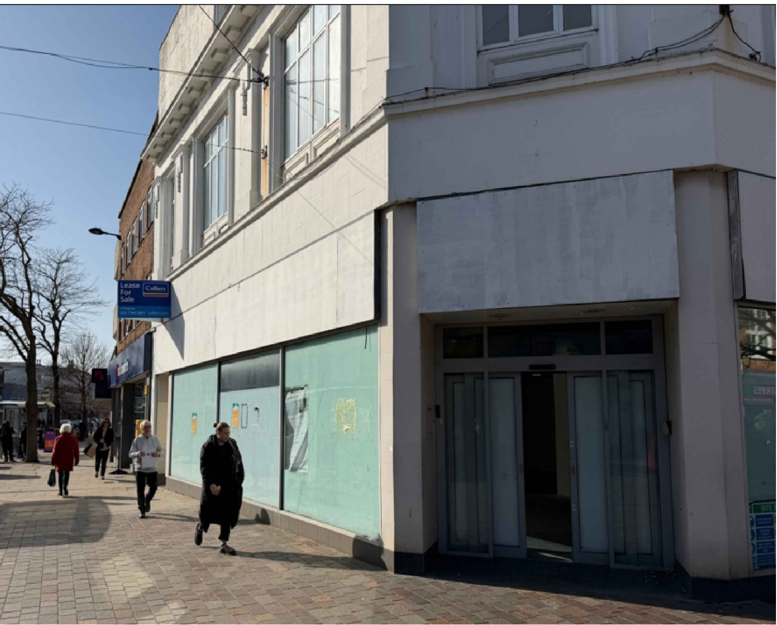
PHOTO OF EXISTING EAST ELEVATION
