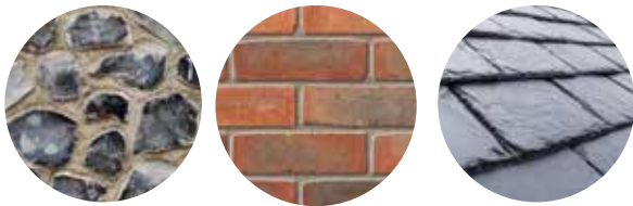
Above: Examples of knapped flint, red multi-brick & grey natural slate roof tiles
