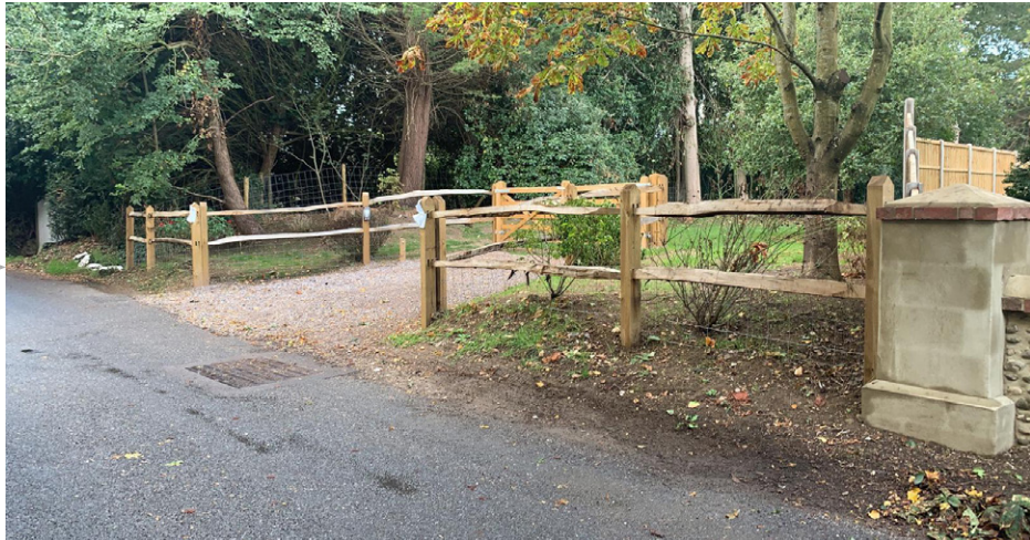
Photograph 4 - Land boundary with Church Lane after the access has been reinstated, looking South West.
