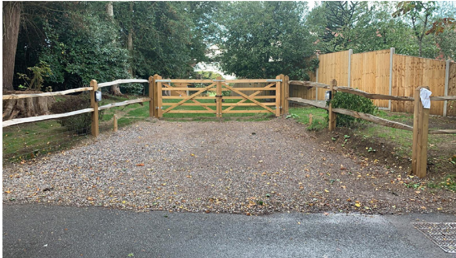
Photograph 5 - Front view of reinstated site access, cleared of scrub/ bushes with some pruning of trees. No trees have been removed.
