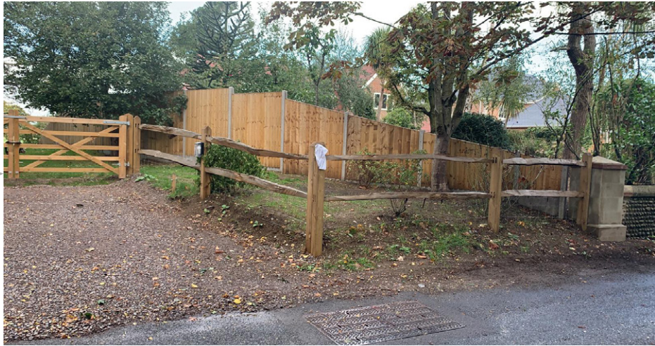
Photograph 3 - Land boundary with Church Lane after the access has been reinstated, looking North East
