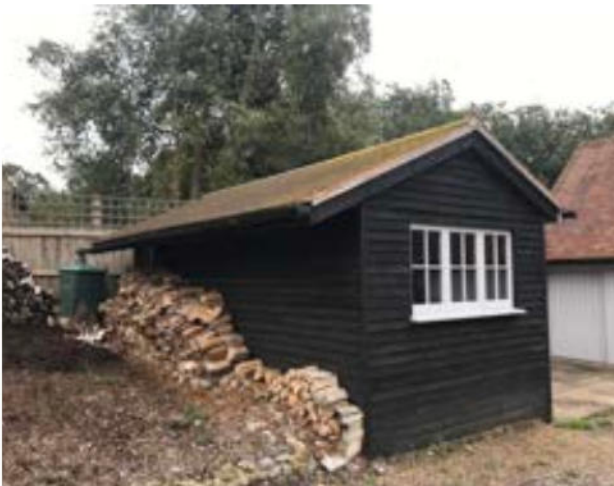
Image 15: Southern aspect of Barn 1.
