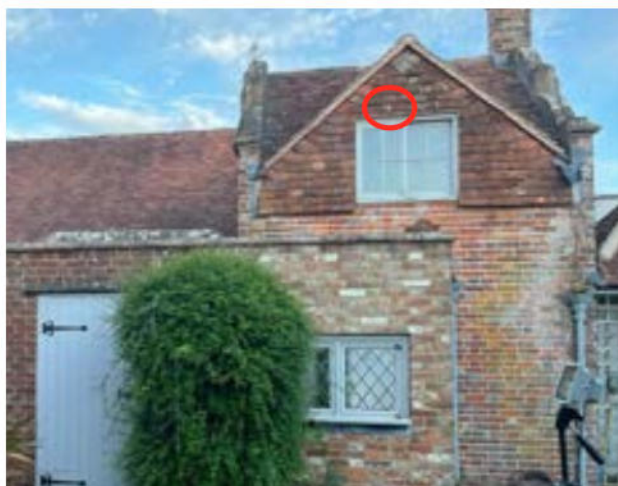
Image 19: Emergence location of the common pipistrelle behind hanging tiles on the western aspect.
