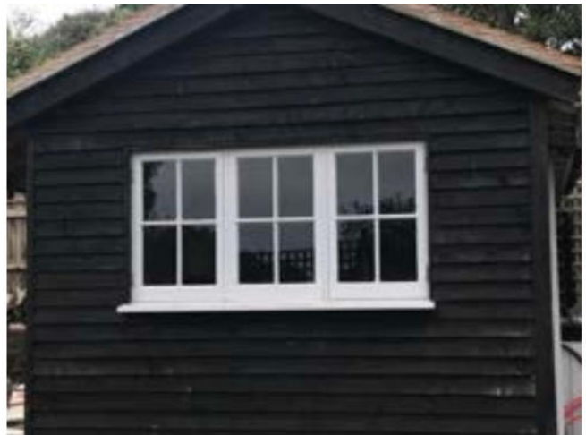
Image 16: Western aspect of Barn 1, where the bat dropping was found.
