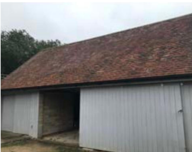
Image 17: Southern aspect of Barn 2.
