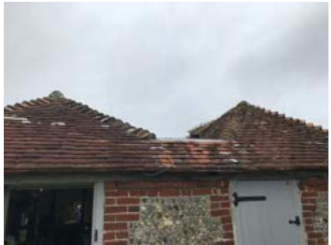
Image 14: The double-pitched roof of the living accommodation.
