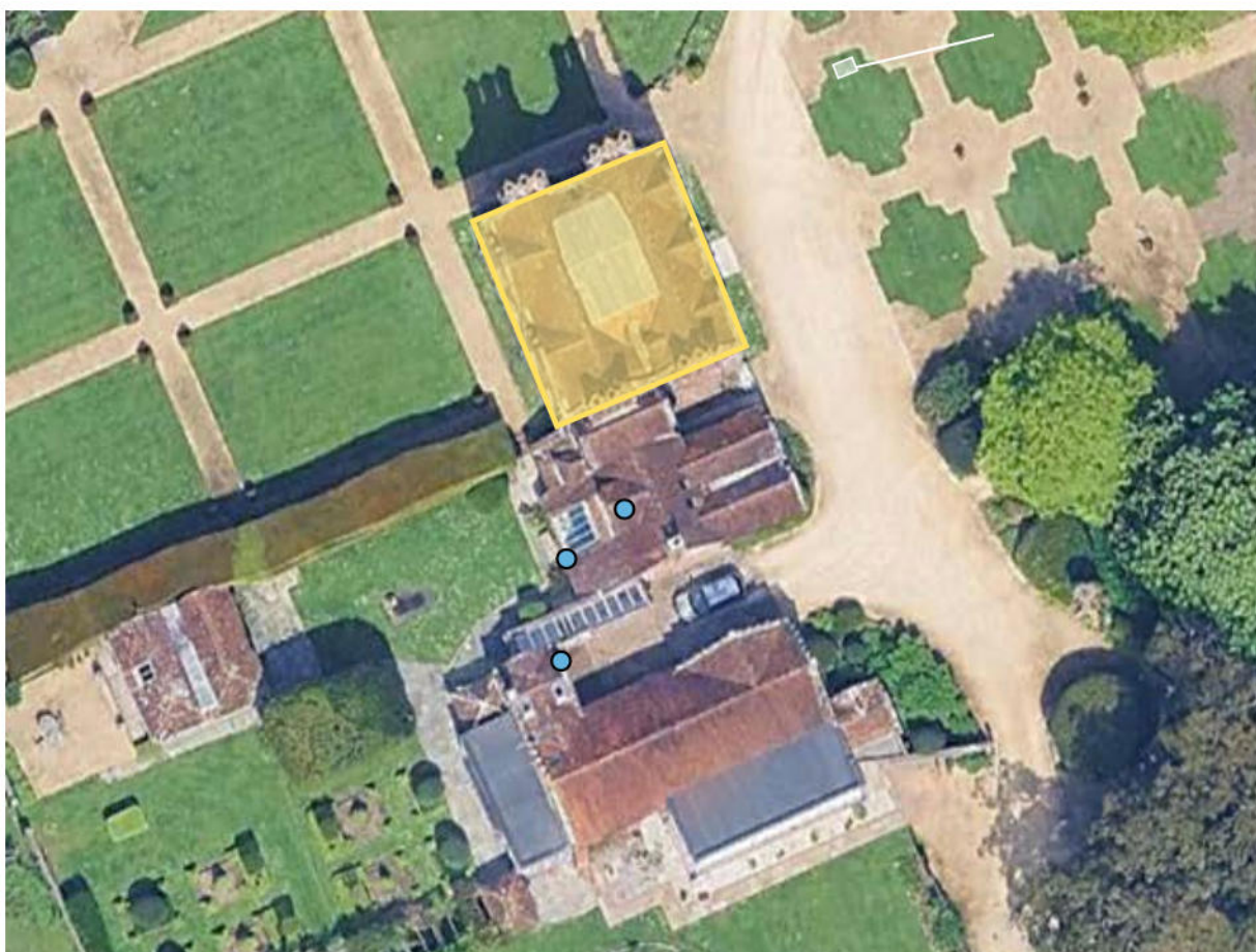
Figure 6: Original house within B1, that requires immediate works, highlighted in yellow. Bat roost locations highlighted with blue circles (Copyright Google Earth Pro, July 2026)
