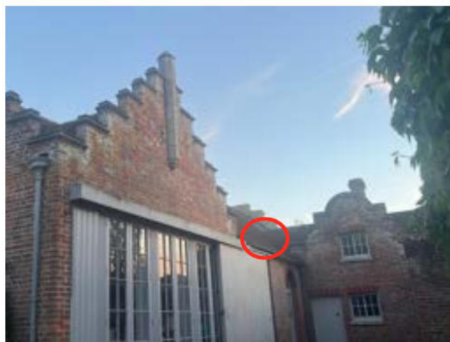
Image 20: Emergence location of the common pipistrelle beneath roof tiles on the eastern aspect.
