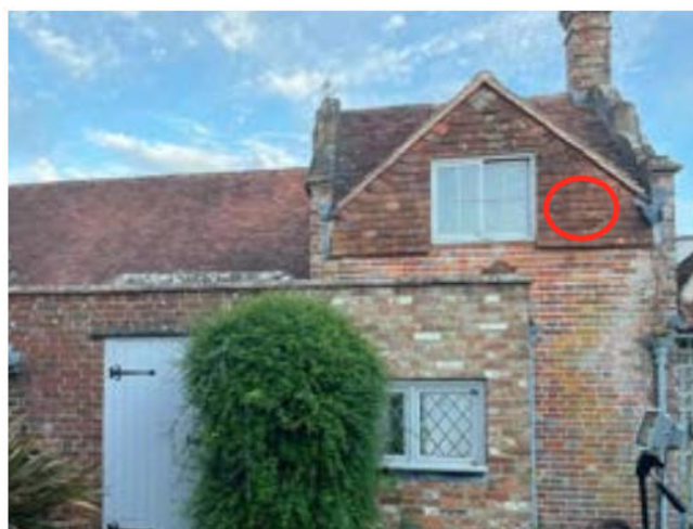
Image 22: Emergence location of the common pipistrelle behind hanging tiles on the western aspect.
