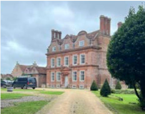
Image 7: The front aspect of the property, showing brickwork in excellent condition.
