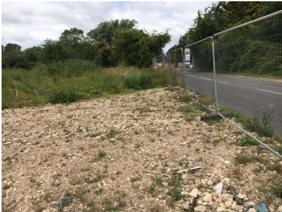
Photograph 2: Compacted ground (north of site)
