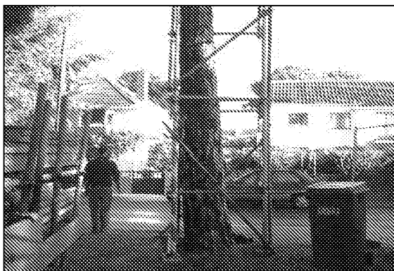
Photo 5: A scaffold braced framework surrounding the trunk reduces the risk of accidental impact.
