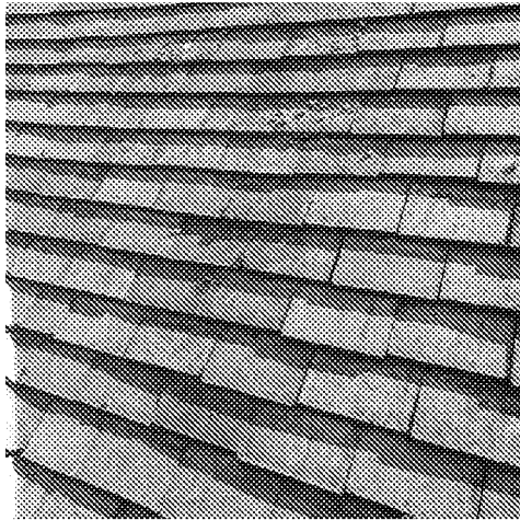
i) Proposed reclaimed plain roof tiles and tile hanging
