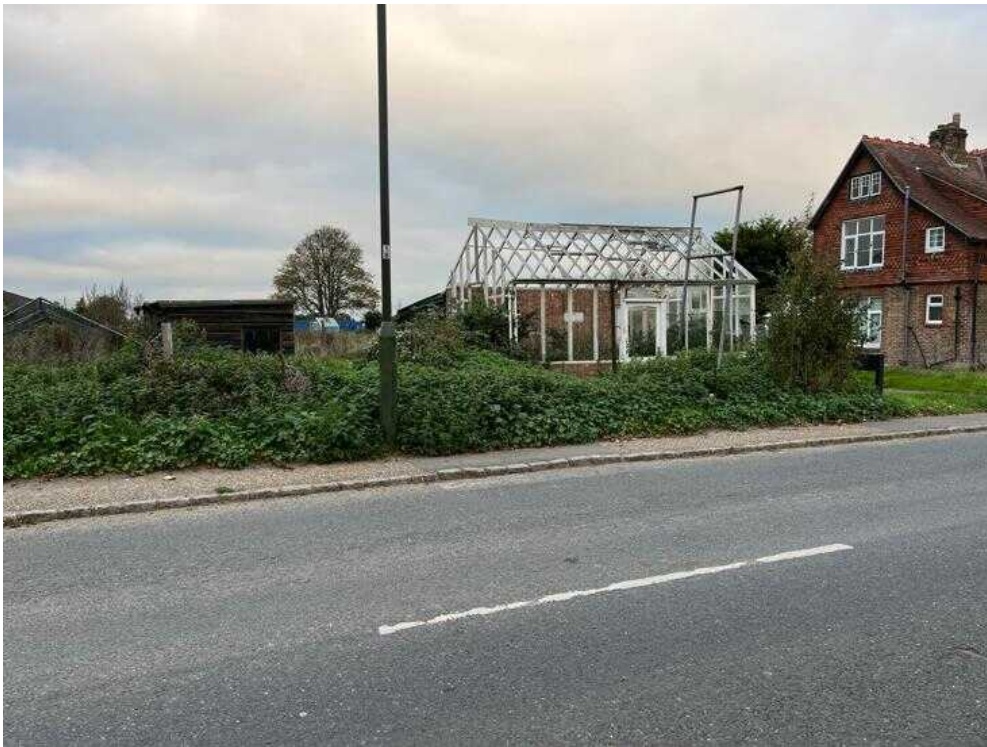
View from the southern side of Yapton Road, looking at the location of the proposed priority junction
