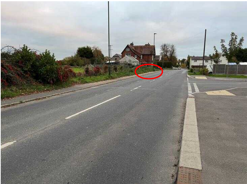
Approaching the site of the proposed priority junction from the east (top) and the west (bottom). The proposed site access is circled
