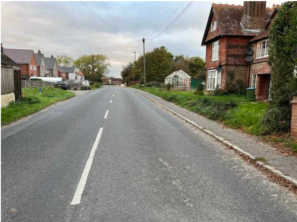
Looking west along Yapton Road. The existing footway on the right is proposed to be widened to 3m to provide shared use and a cycle transition from footway to carriageway
