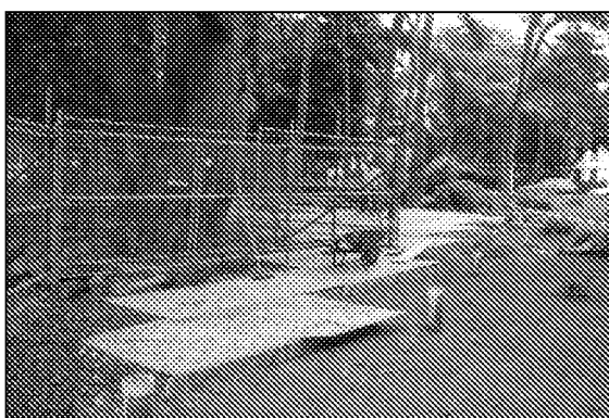
Photo 40: Once the piles have been installed (yellow tops), the ground protection to support the piling rig is removed ready to fix the void-former onto the bare soil, in advance of pouring the building slab.
