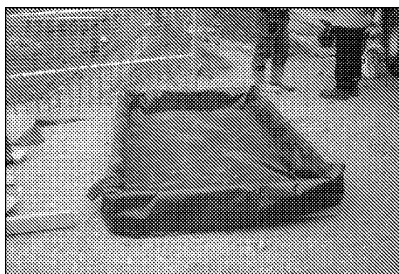
Photo 47: Soil bunding or a supporting framework covered in heavy-duty plastic sheeting is essential where there is a risk of
