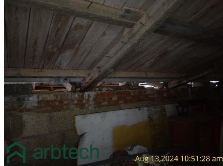
Figure 8- inside access between B3a and B3b
