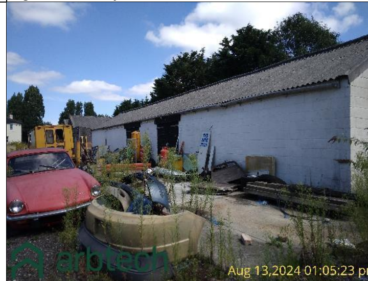
Figure 14-Western view of B5
