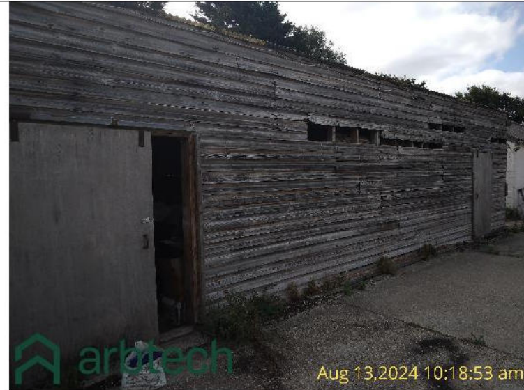
Figure 4, west view of B2
