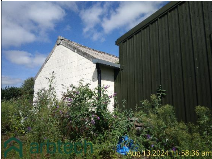
Figure 17- South view of B5
