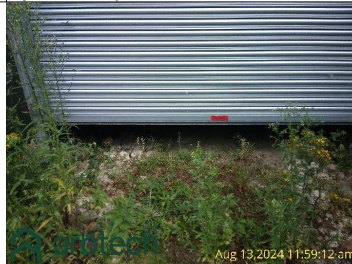
Figure 18-Slightly open door, south elevation of B4
