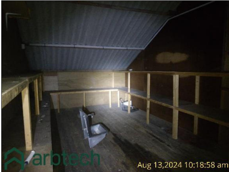
Figure 3- Inside upper loft/room of B1b
