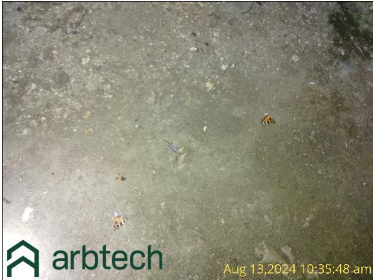
Figure 11- Fresh feeding signs on the floor of B3a
