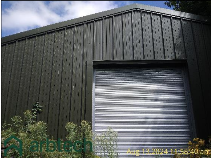
Figure 15- South views of B4
