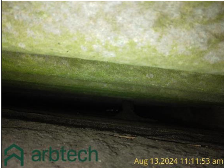
Figure 7- Underneath corrugated roof of B3a
