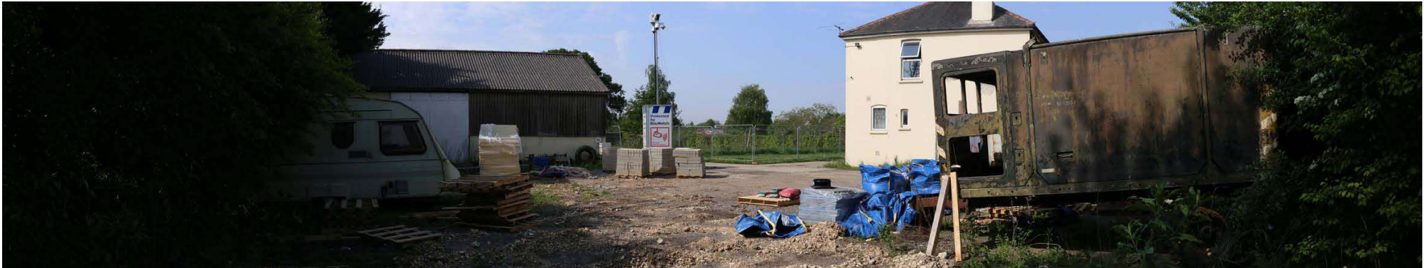
Site Photograph A. South-westerly view from the north-eastern corner of the Site showing various discarded elements adjacent to the white rendered facade and slate roofed Hill View.
