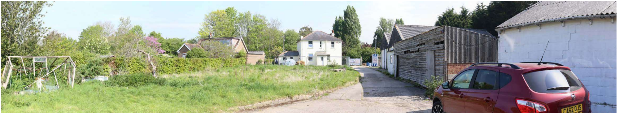
Site Photograph B. A disused industrial park including commercial barn buildings, accessed off Eastergate Lane, from east of Hill View. The curtilage to Hill View extends to north, with native hedgerow to west.
