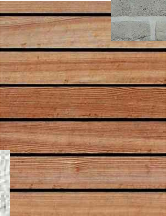
Untreated horizontal Larch timber cladding
