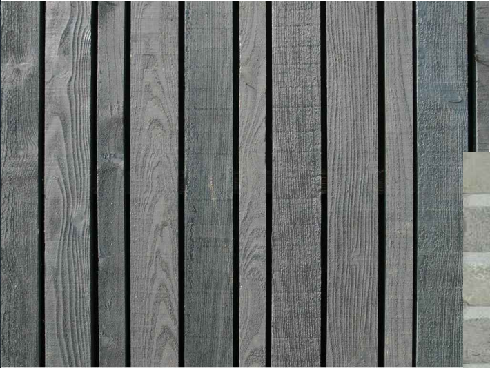
Black painted vertical timber cladding
