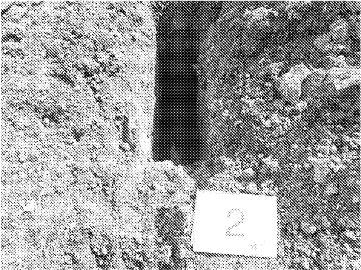
Record Photo of Trial Pit 2
